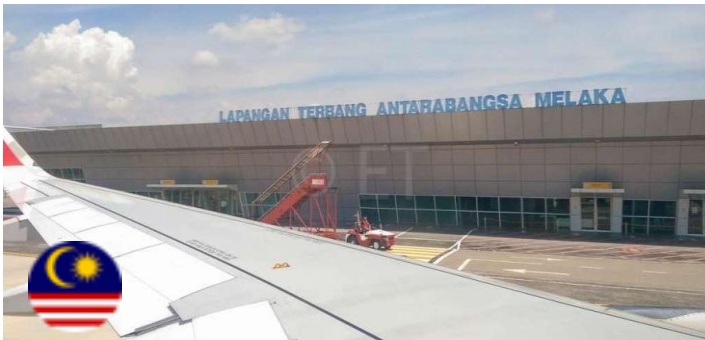
Location: Melaka Airport, Melaka Capacity: 404 kWp Contract: 20 years PPA with Malaysia Airports
