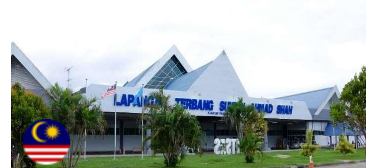
Location: Kuantan Airport, Pahang Capacity: 404 kWp Contract: 20 years PPA with Malaysia Airports
