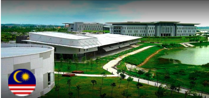
Location: Kampar, Perak Capacity: 4.1 MWp Contract: 21 years PPA with UTAR
