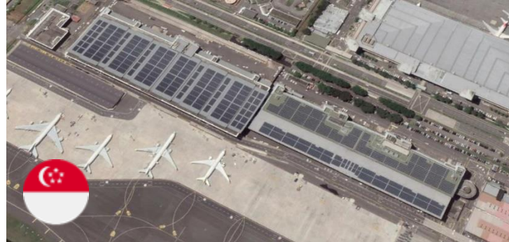
Location: Changi Airport, Singapore Capacity: 3,600 kWp Contract: 20 years PPA with SATS (Divested)
