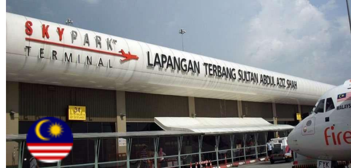
Location: Subang Airport, Selangor Capacity: 1,600 kWp Contract: 20 years PPA with Malaysia Airports
