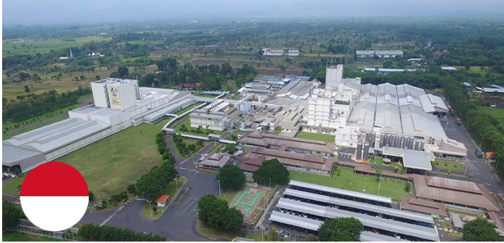
Location: Karawang, Indonesia Capacity: 4.7 MWp Contract: 15 years PPA with Nestle Indonesia
