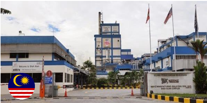
Location: Chembong & Shah Alam, Malaysia Capacity: 1.8 MWp Contract: 15 years PPA with Nestle Malaysia
