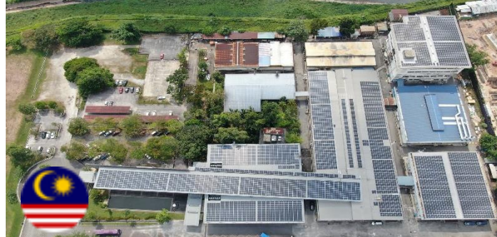
Location: Setapak, Kuala Lumpur Capacity: 1,134 kWp Contract: 20 years PPA with Royal Selangor International
