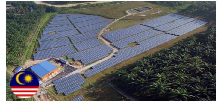
Location: Kuala Sawah, Negeri Sembilan Capacity: 3.30 MWp Contract: EPCC
