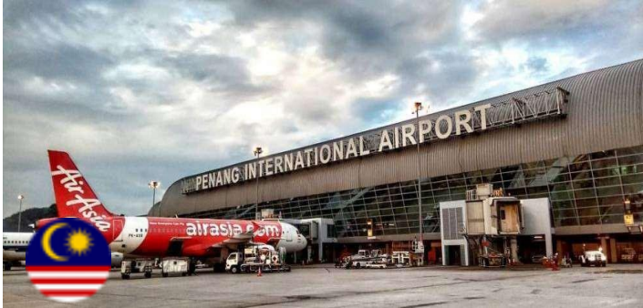
Location: Bayan Lepas Airport, Penang Capacity: 2,600 kWp Contract: 20 years PPA with Malaysia Airports
