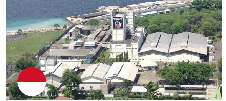
Location: Panjang, Sumatera, Indonesia Capacity: 1.3 MWp Contract: 15 years PPA with Nestle Indonesia
