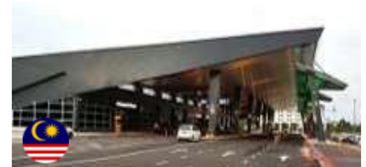
Location: Langkawi Airport, Kedah Capacity: 1,109 kWp Contract: 20 years PPA with Malaysia Airports
