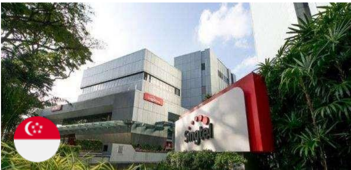
Location: Bedok, Singapore Capacity: 1,652 kWp Contract: 13.5 years PPA with NCS Pte Ltd (Singtel Subsidiary)
